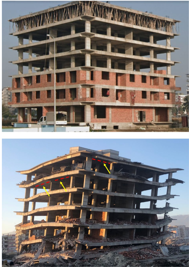
Fig. 8 Building under construction in Hatay (above, Google Maps), and collapsed (below) due to storey mechanism (note also the missing perimeter beams between the columns)
