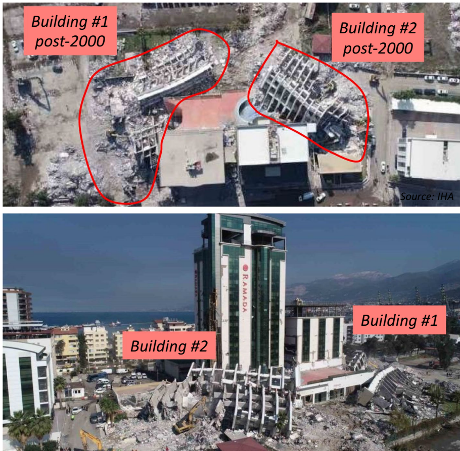
Fig. 11 Two post-2000 buildings collapsed in İskenderun (IHA 2023)
