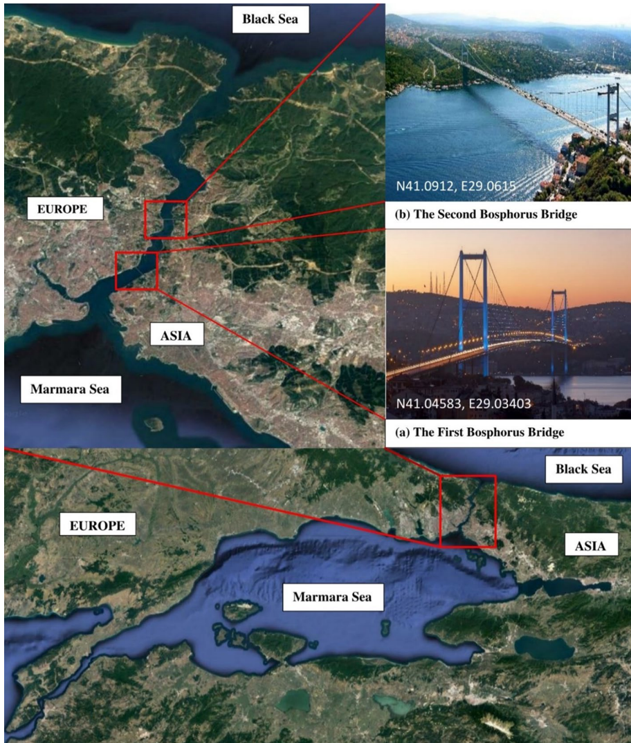
Fig. 2 A general overview and location of long-span bridges: a the First Bosphorus Bridge (the 15 July Martyrs Bridge), b the Second Bosphorus Bridge (the Fatih Sultan Mehmet Bridge)
