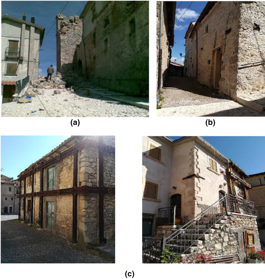
Fig. 6 Typical URM masonry buildings in Rocca di Mezzo and in its sub-municipalities: (a) masonry buildings in Rocca di Mezzo damaged after 2009 L'Aquila earthquake, (b) masonry buildings repaired with horizontal steel ties in Rovere, (c) post-earthquake temporal safeguards applied to masonry buildings in Fonteavignone (photos date back 2021)
