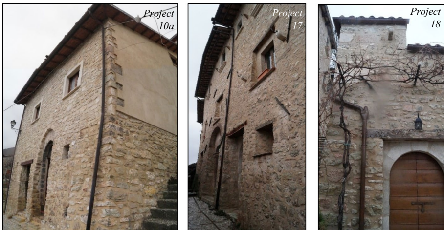
Fig. 18 MSUs, located in Campi Alto, with no external damage and damage index equal to 0 (project 18) or 1 (projects 10 and 17)
