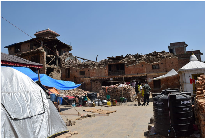
Fig. 13 Structure damage observed at Bungmati village near Bhainsepati—no evidence of liquefaction (Liq. ID 8 in Table 6) [Photo: RM Pokhrel]
