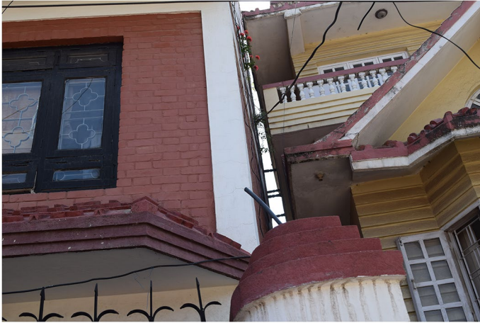
Fig. 12 Tilted building due to liquefaction at Imadol (Liq. ID 6 in Table 6) [Photo: RM Pokhrel]
