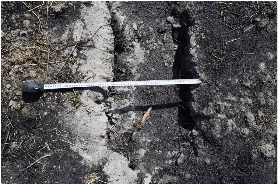
Fig. 11 Liquefaction and sand boiling at Bungmati (Liq. ID 3b in Table 6) [Photo: RM Pokhrel]
