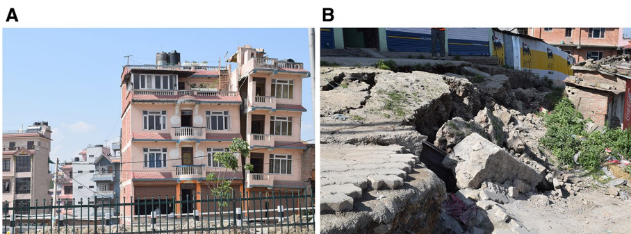
Fig. 5 a Partial collapse due to tilting and seismic pounding in the Kausaltar area (Location 7b in Fig. 2) after the Gorkha earthquake; b liquefaction and cracks in the ground near the Araniko Highway at Kausaltar, Bhaktapur, as a result of the Gorkha Earthquake 2015, (Location 7c on Fig. 2). Photograph taken on 2015-05-31 [RM Pokhrel]
