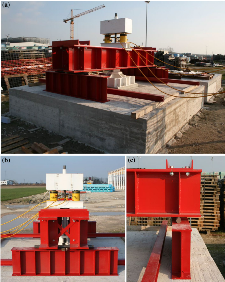
Fig. 12 Setup for tests on anchor groups: a overall view; b front view of test rig; c detail view of one of the supports of the reaction frame
