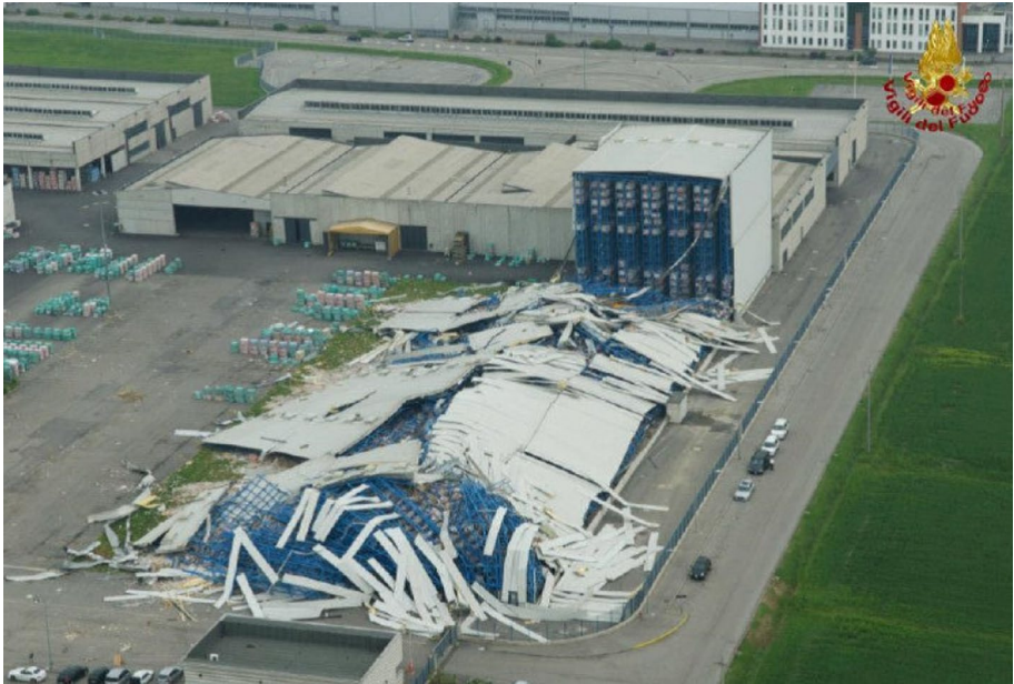
Fig. 1 Aerial view of the struck industrial area showing the collapsed warehouse (courtesy of the Italian National Fire Corps)
