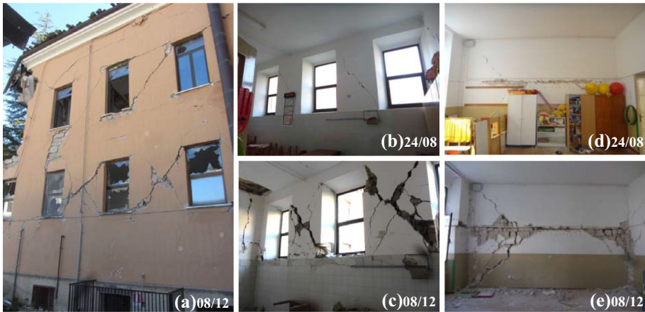
Fig. 6 Photos of P. Capuzi school that testify the occurrence of a prevailing in-plane response (activated starting from 24th August 2016 and then further aggravated after the next shocks): external (a) and internal views (b/c) of Wall 8; internal side wall oriented in Y direction (d/e). The walls numbering refers to that introduced in Annex I-Benchmark Structures Input Data
