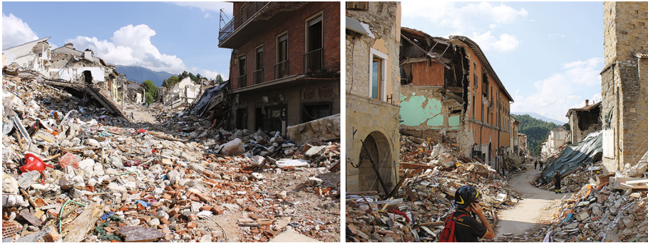
Fig. 11 Overview of damage on Corso Umberto: east (left) and west (right) of Via Roma
