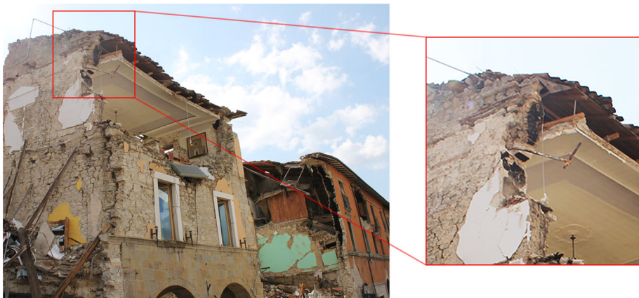
Fig. 14 Partial facade collapse (mechanism M3) of a building which had tie rods: general view (left) and detail (right)
