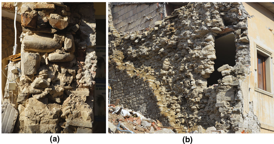
Fig. 18 Example of ev4 vulnerability factor (poor quality masonry): a absence of bondstones in the wall-section; b cobblestones with poor quality mortar
