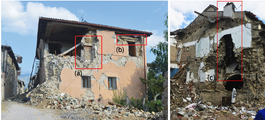
Fig. 19 Example of ev12 vulnerability factor (local discontinuities): closure of previous wall openings (a), presence of weak wooden elements (b), presence of chimney in the wall (c)
