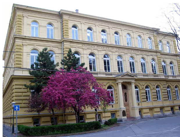
Fig. 4 The building of the 1st Department of Pathology of the Semmelweis University, Budapest. Photo: Mária Cserneký 2008 (reproduced with the permission of the copyright holder)
