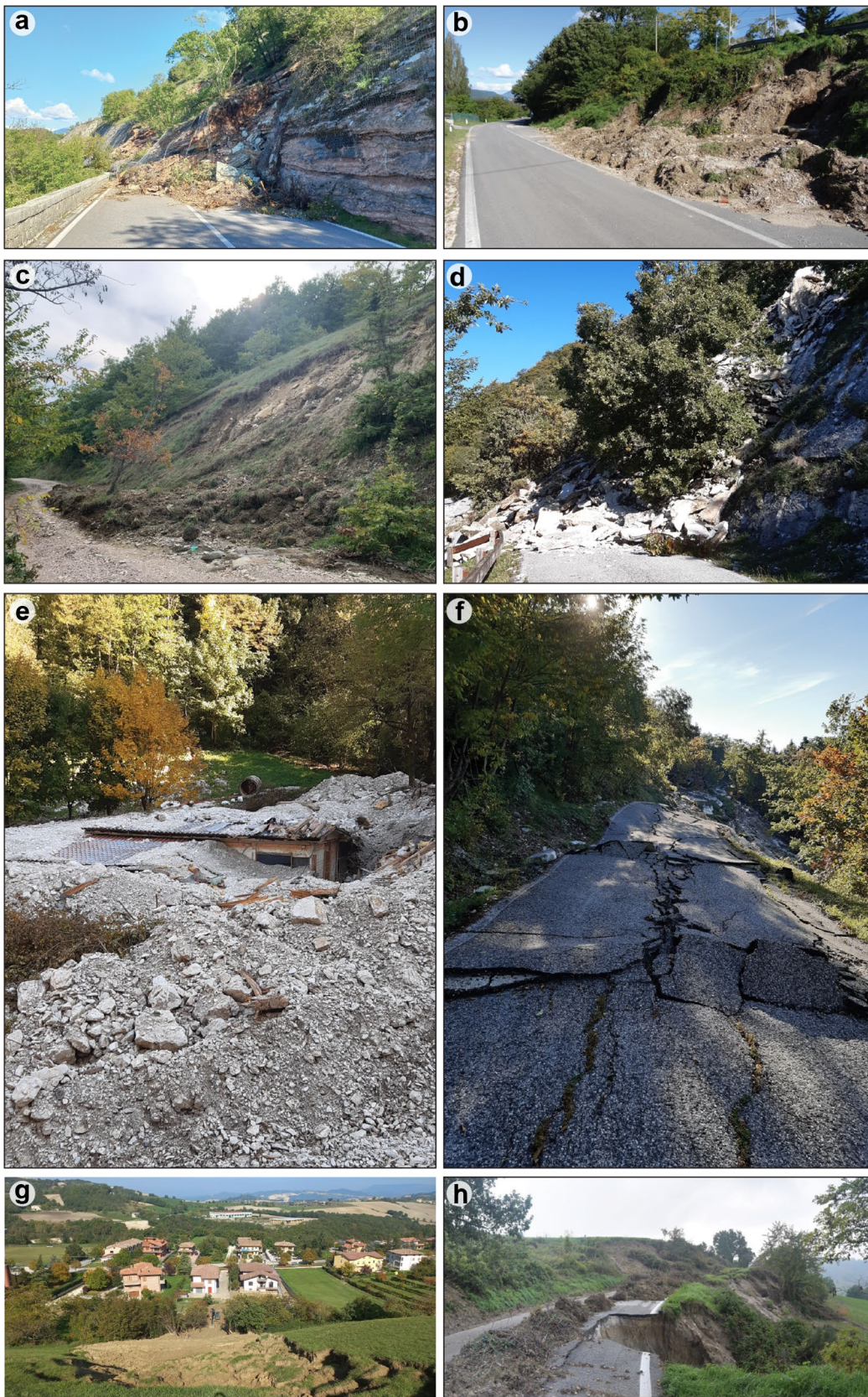
Fig. 5 Examples of landslides that hit roads and structures. a Rock slide on the SS3 national road, Scheggia municipality; b, c, h, g earth slide; d rock fall; e debris flow; f rock slide
