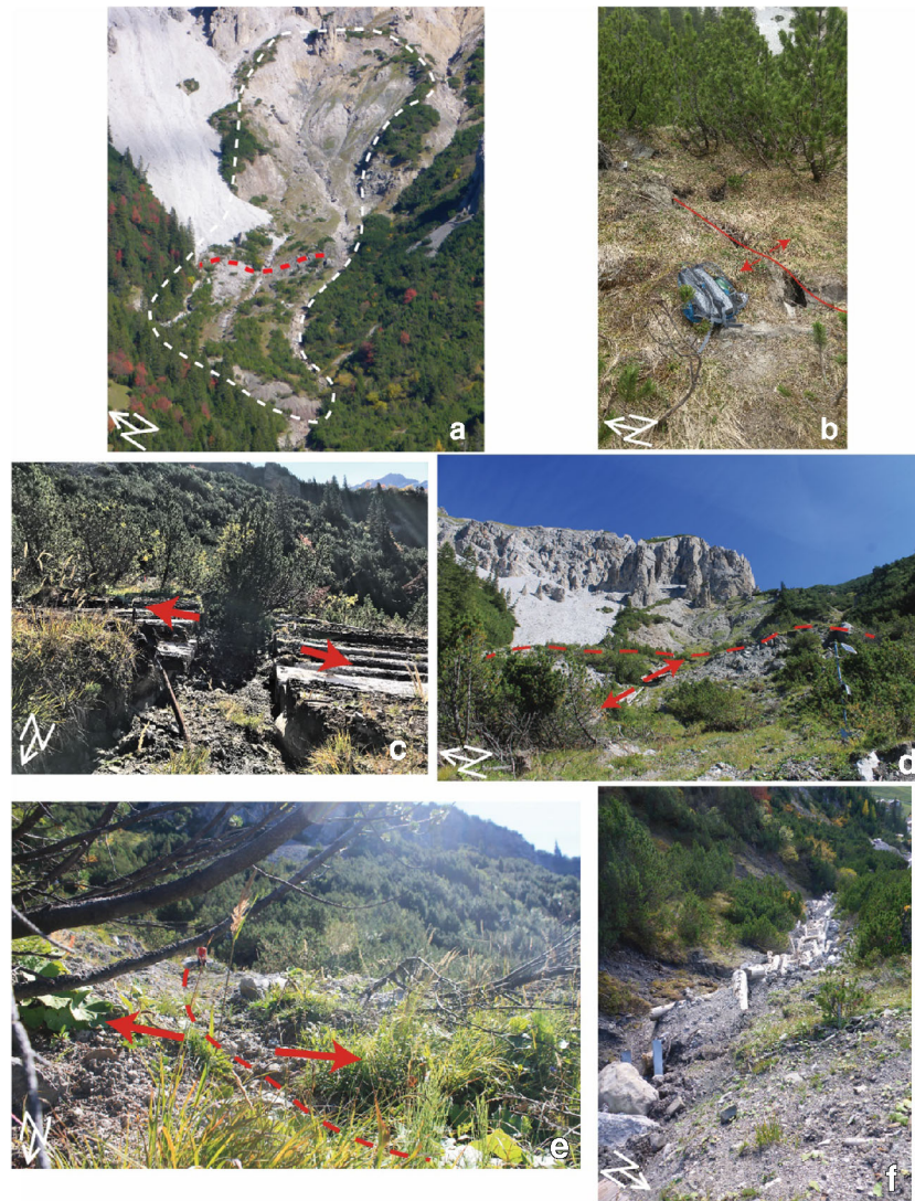
Fig. 4 a Oblique view of the landslide body, showing the landslide outline (white line) as well as the backscarp that formed after 2015 (red dashed line). b Image of a linear extension feature near the toe of the landslide. c Landslide surface drainage system that has undergone extension. d Backscarp of the landslide and damage to the surface drainage system. e Linear internal deformation feature showing extension. f Damage to the surface drainage system on the left flank of the landslide. The locations where images b, d, e, and f were taken are shown in Fig. 2
