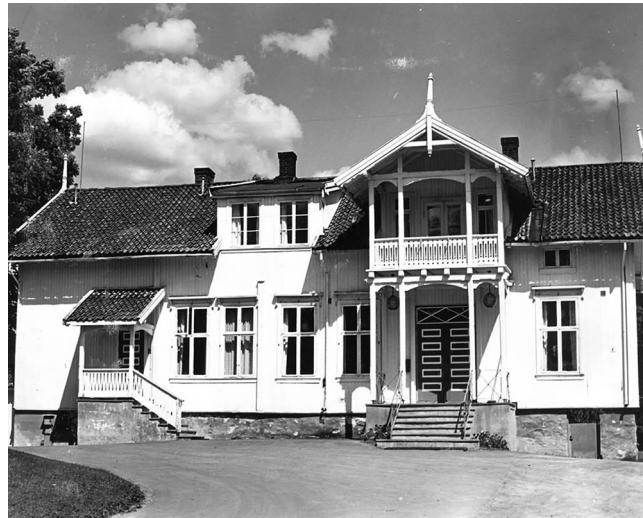
Fig. 4 ◀ The main house of the farm after the conversion into an epilepsy colony
