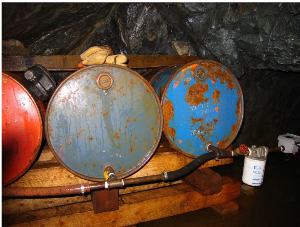
Fig. 1 Ethylene glycol feed drums, connected to a filter and battery-operated and timed drip system (photo by A. Sobolewski)
