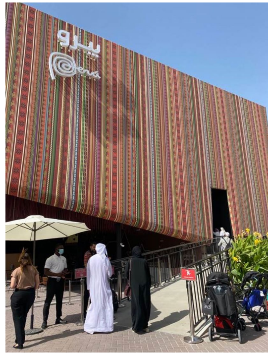
Fig. 11 Ramp access to the Peruvian pavilion
