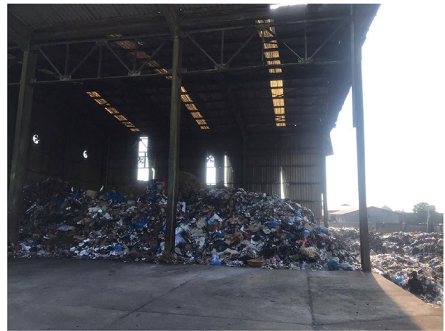
Fig. 8 Showing the waste transfer station in Liberia
