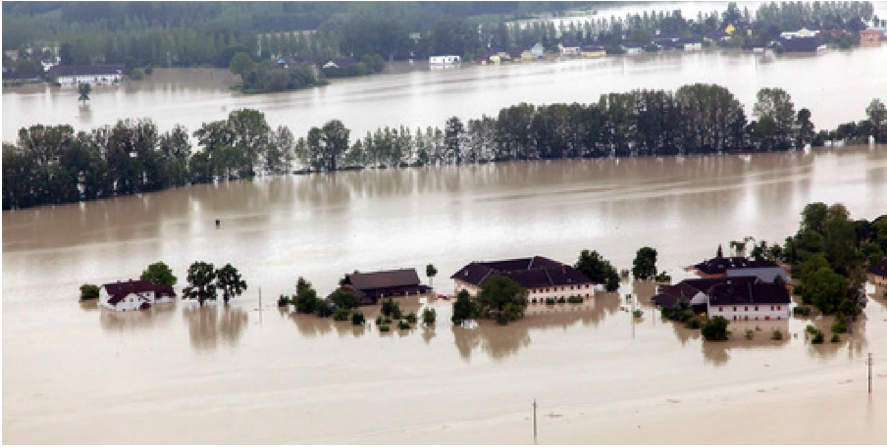
Fig. 4 Flooded village in Eferding Basin 2013. Image source: police records
