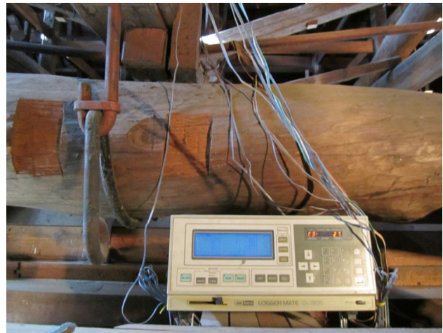
Fig. 3 Measurement of strain associated with dismantling
