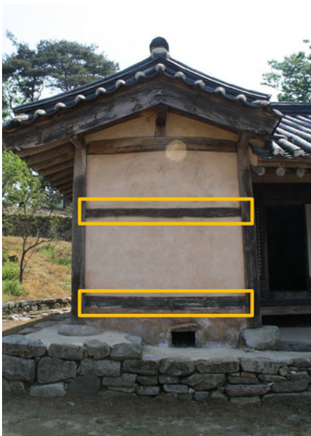
Fig. 1 Middle and bottom lintel in Han-ok
