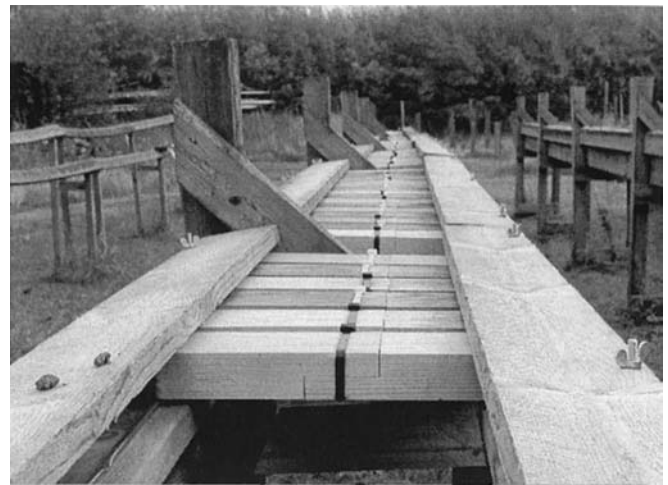
Fig. 2. The body of the lap-joint and the joint in the middle of the unit
