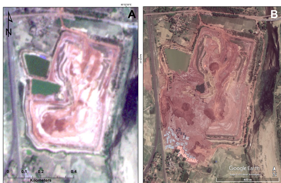
Fig. 12 A Pre-failure (9 April 2019) and B post-failure (9 May 2019) satellite images of the 9 April 2019 Hindalco tailings dam breach in India. Image A is PlanetScope (3 m resolution) and image B is Google Earth Worldview-2 (0.5 m resolution)
