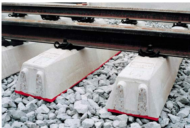
Fig. 1 Ballasted track with under sleeper pads
