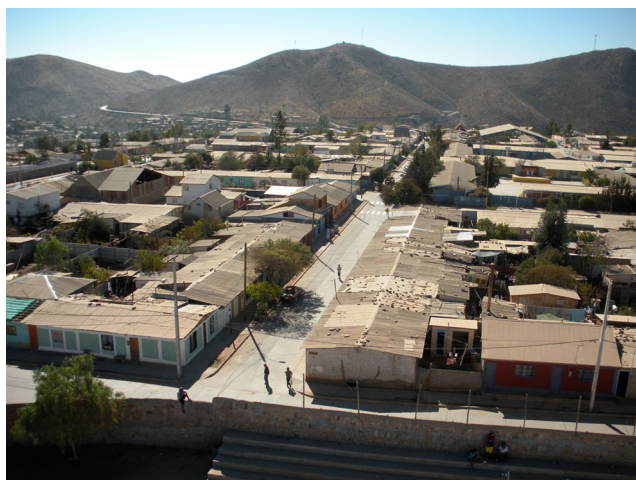
Fig. 1 Photo of Andacollo study area during April 2009 from approximately 20 m a.g.l. View is towards the north. The location of the photo is shown in Fig. 2
