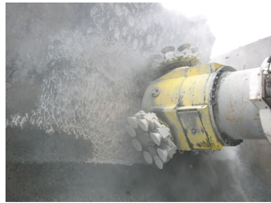
Fig. 28 The new generation mining head with disc tools during field tests
