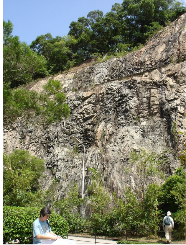
Fig. 4 The Chinese University rock cut slopes, Hong Kong
