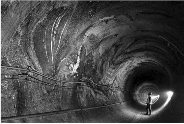
Fig. 14 Folded and faulted (ductile) ground in the Glendoe high race tunnel—well away from the Conagleann Fault Zone (BGS photo)
