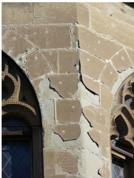
Fig. 1 Contour scaling pattern developing on Villarlod molasse at the Fribourg city hall
