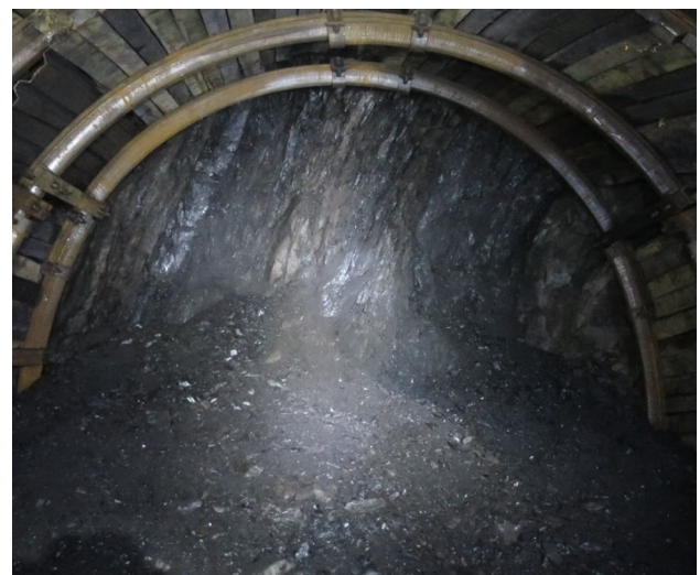
Fig. 3 Sublevel development heading in Seam #8 illustrating the friable nature of the coal seam
