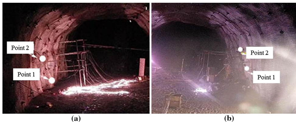
Fig. 14 Location of the selected points for PPV and displacement measurements in a Test 1 and b Test 2
