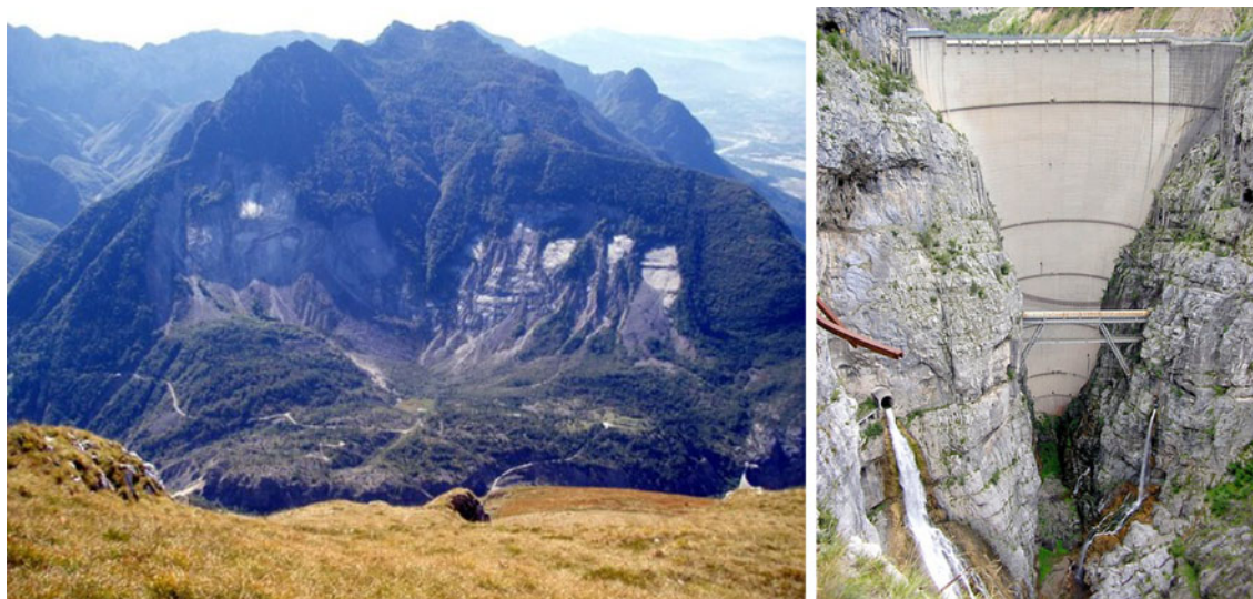
Fig. 1 Panoramic view of the slip surface of the Vajont landslide and of the double curved arch dam
