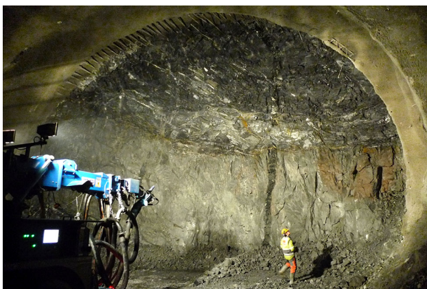
Fig. 6 Typical geology of intrusions. Sub-horizontal syenite intrusion and steep diabase dyke in sandstone (top) at profile no. A1239
