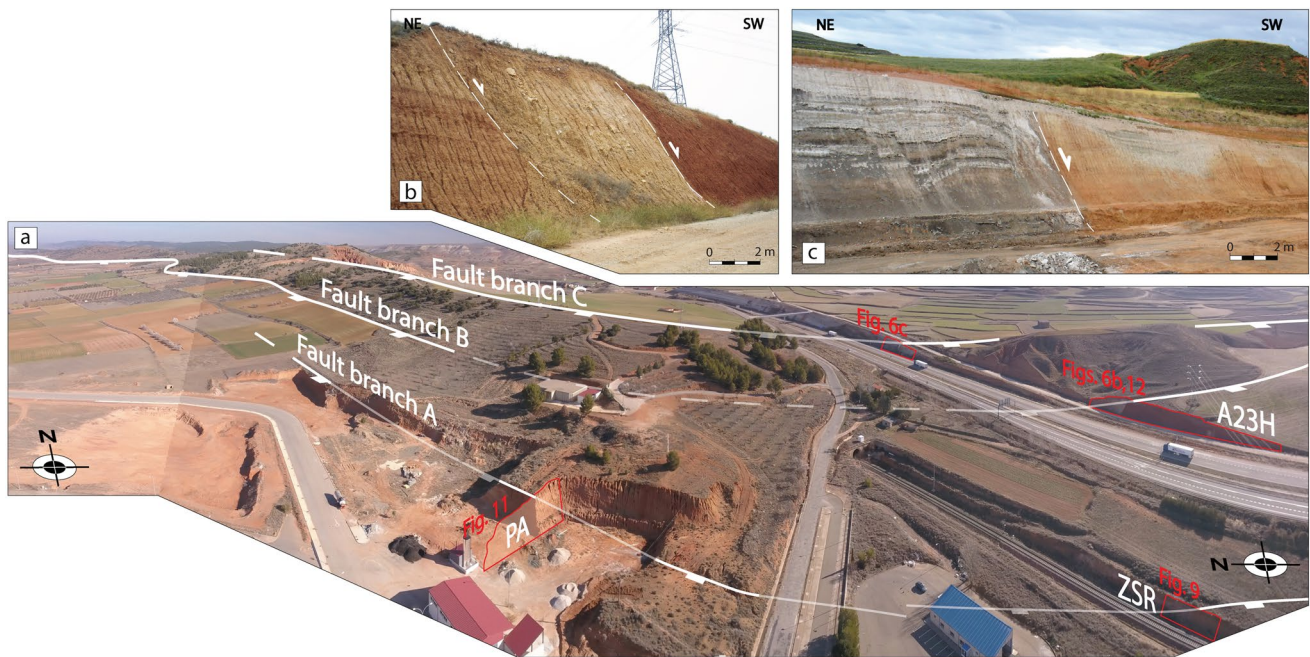
Fig. 6 a Oblique aerial view of the area east of Calamocha town, where the traces of fault branches A, B and C representing the central sector of the Calamocha fault zone are drawn. b Branch B exposed
