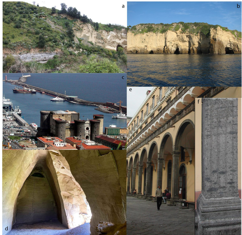
Fig. 6 The Neapolitan Yellow Tuff and Piperno (CI unit) deposits, which were extensively quarried, and buildings they were used to construct. a The Piperno (grey truncated unit in lower left of image) and NYT deposits (upper right) in the Verdolino Valley along the NE edge of the caldera. b A NYT exposure in the Posillipo cliffs, on the eastern margin of the caldera. c The mediaeval Castel Nuovo of Naples (also known as Maschio Angioino) that was built in 1279 CE from both the NYT (walls) and Piperno (towers) deposits. d NYT as it appears in the San Rocco (Naples) quarry. e The Piperno (CI) facies is used in the San Marcellino building in central Naples, and f noticeably for the columns
