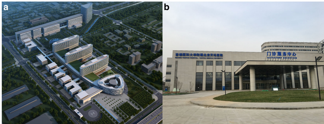
Fig. 6 Cover figure. Computer graphic of the brand-new Beijing Tiantan Hospital building (a) and its outpatient clinic now under construction (b), which opened at the end of 2017. New facilities have replaced the old wards at a new address
