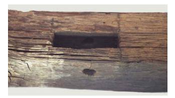
**Fig. 11** Indications for secondary use on a bridge element; nonfunctional cross connection and part of a tenon and mortise joint (photo Archeologisch Centrum Leiden/BIAX *Consult*)
