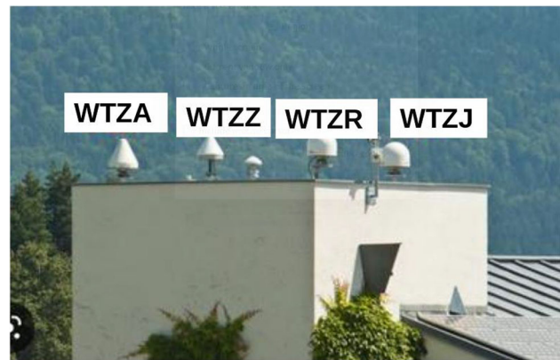
Fig. 3 Location of four GNSS stations in Wettzell, Germany, courtesy from the EPN website
