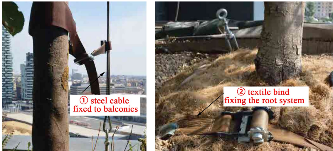
Fig. 5 Artificial mechanical anchoring of trees on balconies in Bosco Verticale (Giacomello 2015)
