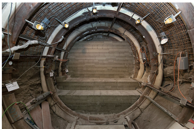
Fig. 17 Photo (by COMET) of the unfinished bentonite block wall in the ‘interjacent sealing section’ (ISS) at the deep end of the FE tunnel
