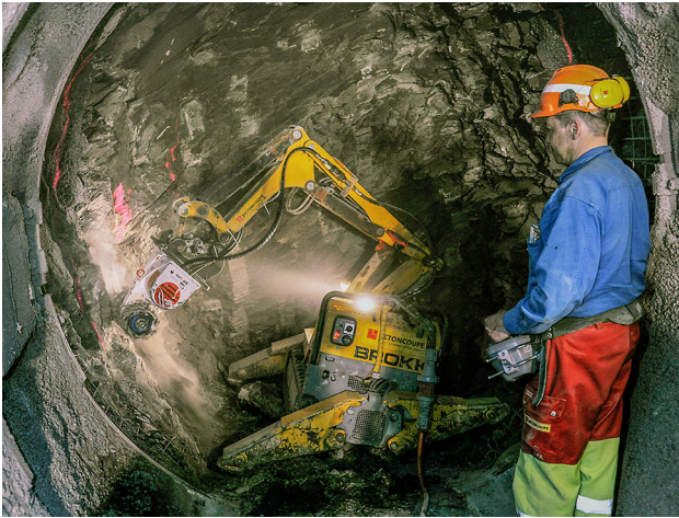
Fig. 2 Photo (by COMET) of the excavator (equipped with a small rotary drum cutter) used in the FE tunnel mainly for profiling
