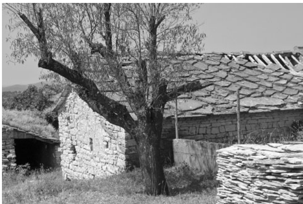
Fig. 2 Pile with slabs of platy limestones of the Benovac Stone, and in the background an old house roofed by the same rock. Benkovac, Croatia
