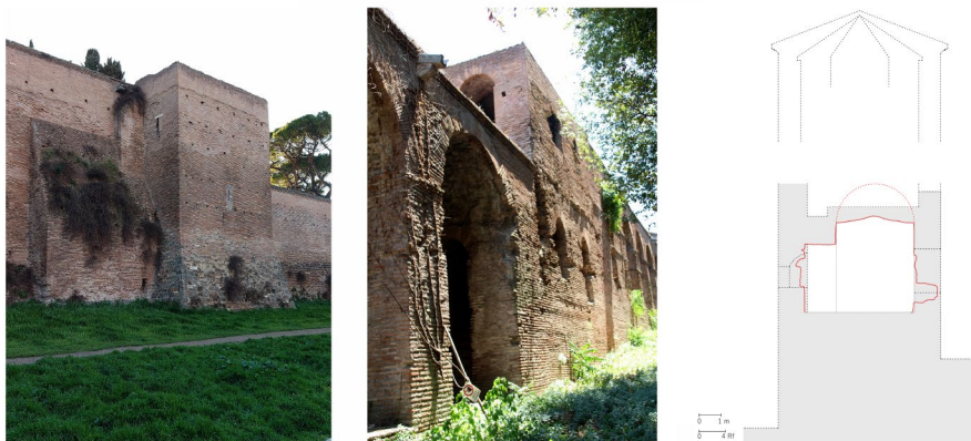
Fig. 3 Views of the tower J17 from the exterior (a) and interior (b) side of the Walls; (c) Section of the vault with reconstruction of the tower based on Vitti hypothesis. Image: authors based on Vitti 2013: 140
