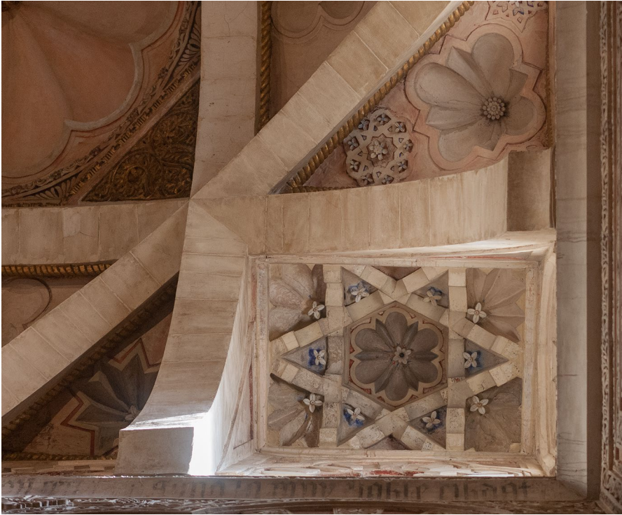
Fig. 20 Vault over the first bay of the central nave of Al-Hakem II in the Great Mosque of Cordova. Detail of rib intersections. Image: author
