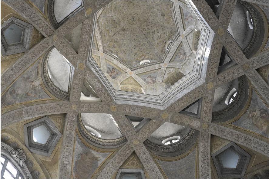
Fig. 19 Main dome in San Lorenzo in Turin. Detail of rib intersections. Image: author
