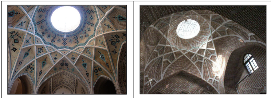
Fig. 3 Examples of Plumb Karbandi. a Left Men's bathroom of the Kashan Āmeri House, b right Haj Safar Ali Mosque in Tabriz
