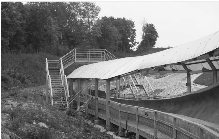
Fig. 4 Bobsleigh track in Paramonovo, Moscow region. Above the radial cross section in the highest point of the curve. Author's original contribution. Below pedestrian bridge overpass. Author's photo, August 2010
