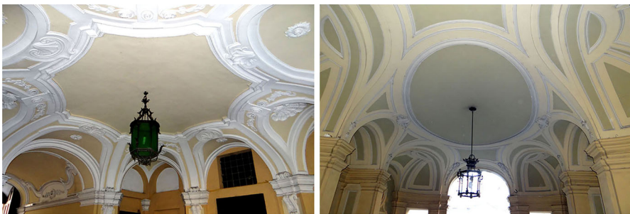
Fig. 12 Cases in which the parametric model does not adequately represent the characteristics of the vaults. This occurs when the atrium has a different plan diagram (via Garibaldi 28—Palazzo Fontana di Cravanza, attributed Plantery) or/and when the angular vaults have a significantly higher level of complexity (via Carlo Alberto 32—Palazzo San Martino di Parella). Photo: Author
