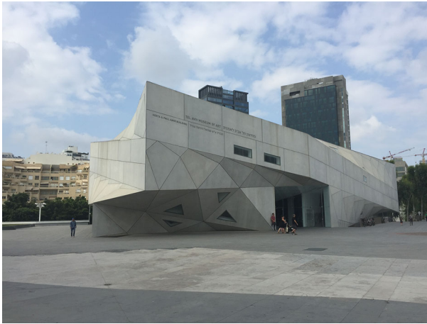
Fig. 1 Tel Aviv Museum of Art, the Herta and Paul Amir Building. Architect: Preston Scott Cohen
