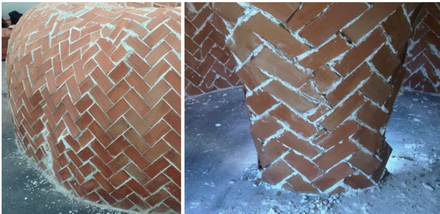
Fig. 1 The free-form dome constructed with non-regular bricks during the 2013 Computational Morphogenesis Workshop held at the Politecnico di Torino
