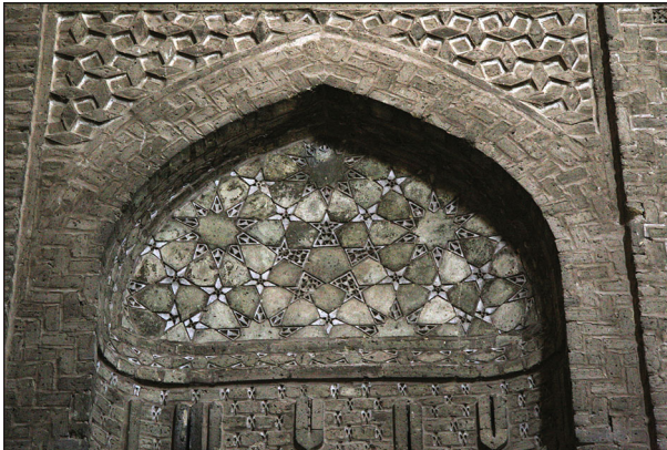
Fig. 32 A 5-fold acute hybrid pattern from the recessed arches in the northeast dome chamber of the Friday Mosque at Isfahan
