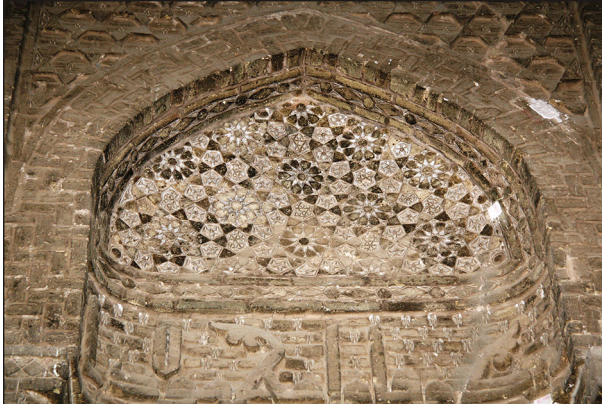
Fig. 30 The classic 5-fold obtuse pattern from the recessed arches in the northeast dome chamber of the Friday Mosque at Isfahan
