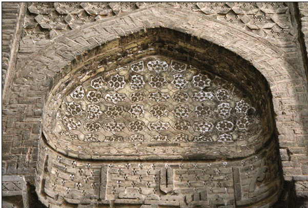
Fig. 28 An orthogonal pattern with 8-pointed stars and octagons from the recessed arches in the northeast dome chamber of the Friday Mosque at Isfahan
