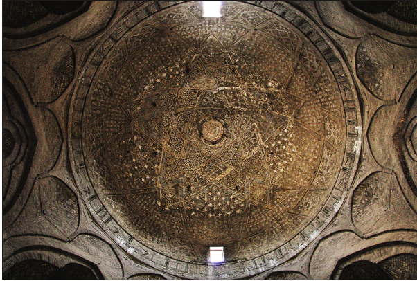
Fig. 38 The dodecahedral 2-point pattern on the dome from the northeast dome chamber of the Friday Mosque at Isfahan
