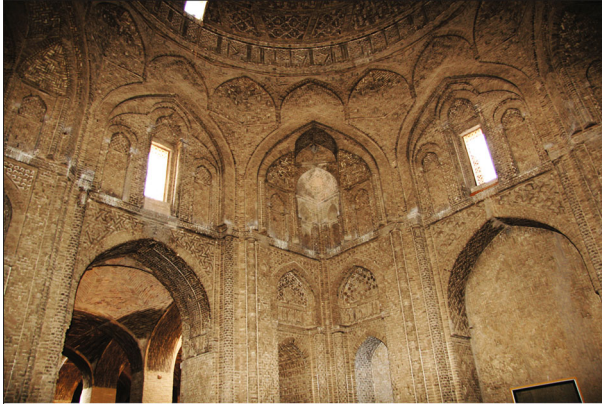
Fig. 6 Recessed arches in the lower portion of the walls of the Seljuk northeast dome chamber in the Friday Mosque at Isfahan
