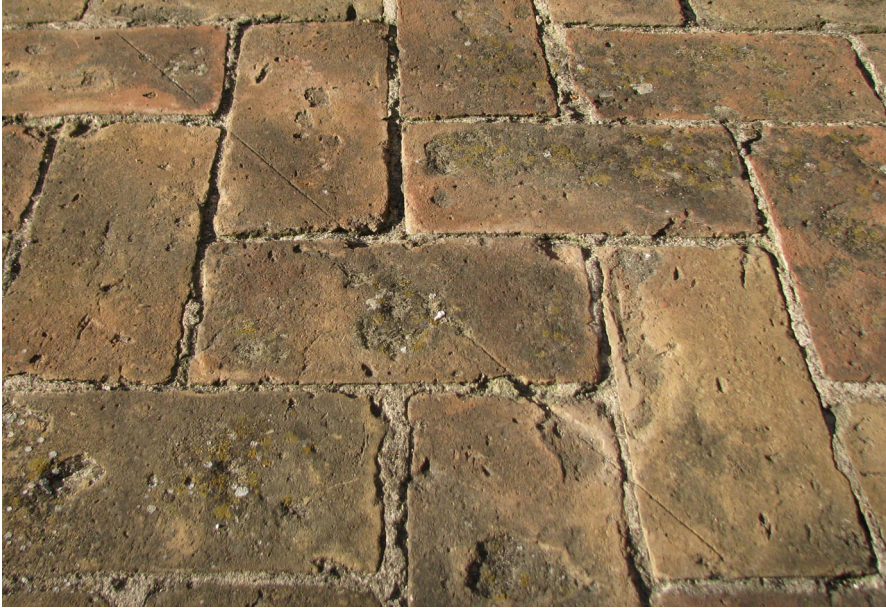
Fig. 6 Detail of the incisions made in the roof bricks. Photograph by the authors
