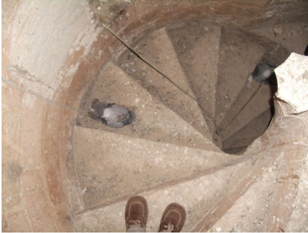
Fig. 5 Helical staircase by tangent solution. Monastery of Santa Cruz la Real in Segovia (Spain)
