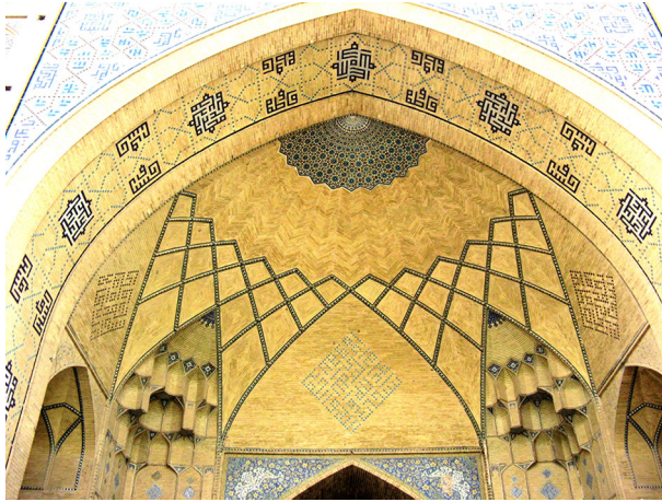
Fig. 32 How can the visitor of this building identify this karbandi using the new method?
