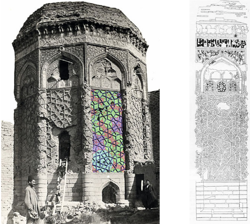
Fig. 10. Gonbad-e Qabud, Maragha, Iran. a) Pattern with pentagonal and decagonal symmetries around shaft of tomb tower, with 'girih' tiles highlighted in one panel [Lu and Steinhardt 2007a: S6 after photo by A. Sevruguin; reproduced with permission of P. Lu]; b) Drawing of one face (after Dastur Corp.) reproduced in [Daneshvari 1982: fig. 128]
