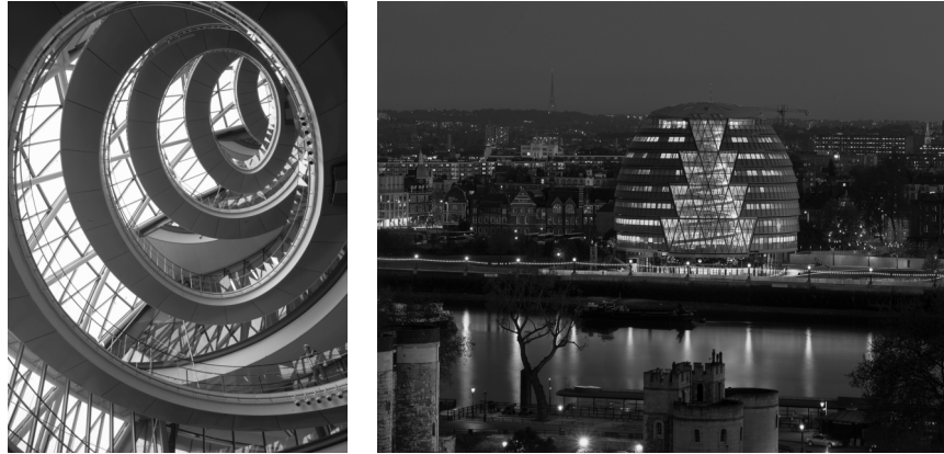
Fig. 3. The conic ramps of London City Hall. Photos courtesy of Foster and Partners
