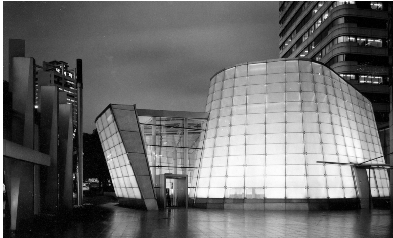
Fig.10. Rodin Museum, Samsung Headquarters Plaza – Seoul (South Korea) by Kohn Pedersen Fox Associates (photo by T. Hursley)
